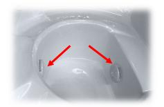
**32.** Once most of the water has been removed, while still blowing, block one of the drains with the plug until there is no more water, then alternate with the second drain. Once there is no more water, blow antifreeze from the filtration until it comes out of both drains and close it with the rubber plugs (**G.**) and make sure that the rubber is flush with the jet and that the wing nut is vertical, tighten it firmly.
