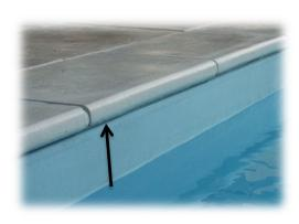
A properly installed coping won't lift off, even if the water level in the pool is higher and the ice applies pressure when it expands.
